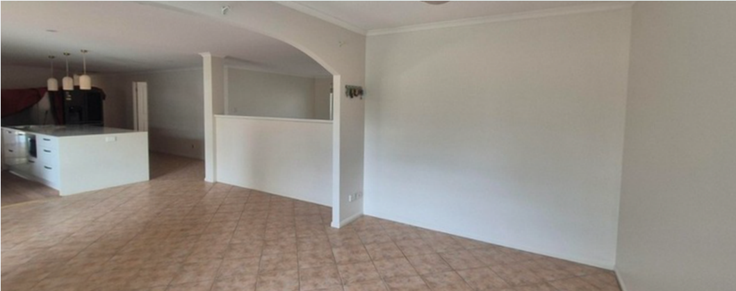
Repair- Ready Handover
